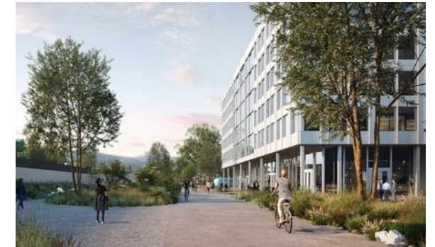
Construction site 3: 13,760 m2 commercial space
